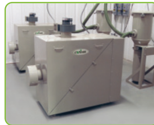
5 HP Pumps in Sound Enclosures
